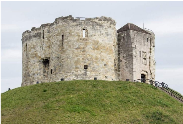
Above: Before works commenced.
