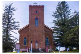
St Thomas Church, Port Macquarie, NSW (1826). This church, built by convict labour from hand-made bricks has suffered foundation movement leading to instability at the corners. Following foundation stabilization, Cintec anchors up to 4 m long have been used to restore the strength of the corners of the building.
