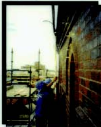
Cintec Anchors Being Carefully Positioned
