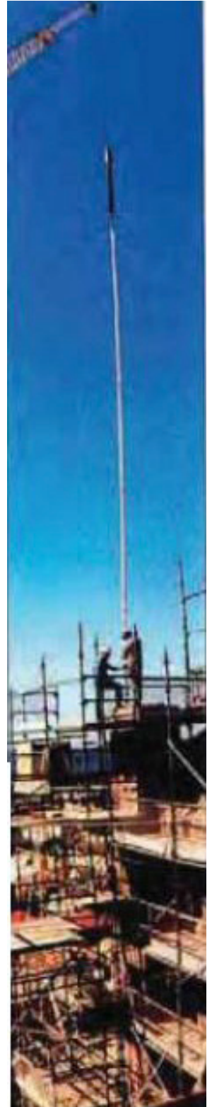
20 m vertical anchor being placed by crane in the project which saw anchors up to 32 m horizontally, Cintec's longest to date.
