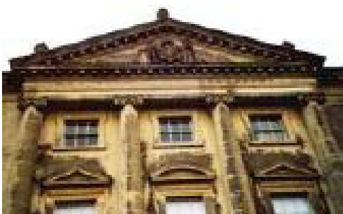
External upper beam area
