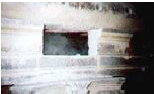
Openings cut in masonry to expose defective wooden beam prior to its removal
