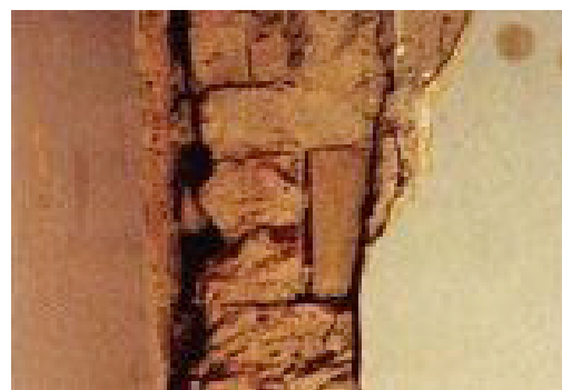
Internal damage of wooden beam
