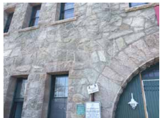
Fig. 11: Completed work before final wash-down
