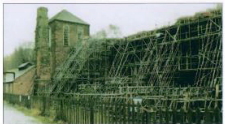
Restoration work in progress
