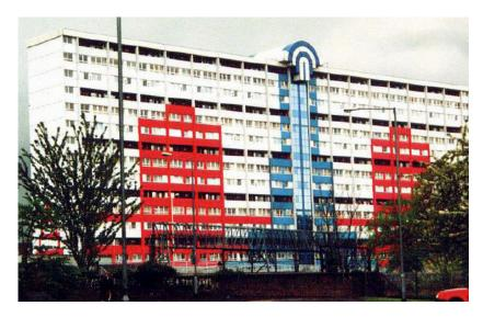
Cintec anchors provide a solution which fixed the external panels to one another and also to an inner wall via the insulation cavity of the hollow concrete flooring. Extensive insitu load testing on the 33.4 mm diameter, 7000mm Long stainless steel tube anchors proved a loading of 240Kn was possible, more than double the 105Kn required strength.
