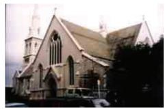
◀ St Philip's Church, Sydney, NSW (1856). Roof spread had led to wall cracking at eave level. Cintec anchors provided the economical repair solution with a guaranteed long life with no visible affect on the building.
