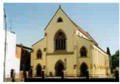
◀ Methodist Church, Maitland, NSW (1858). This building suffered danmage in the 1989 Newcastle earthquake. 6 m Cintec anchors were used in the wall buttresses to provide the additional strength required to resist future seismic damage.
