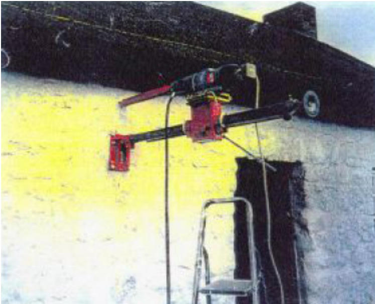
(c) Drilling one of two 60mm holes.
