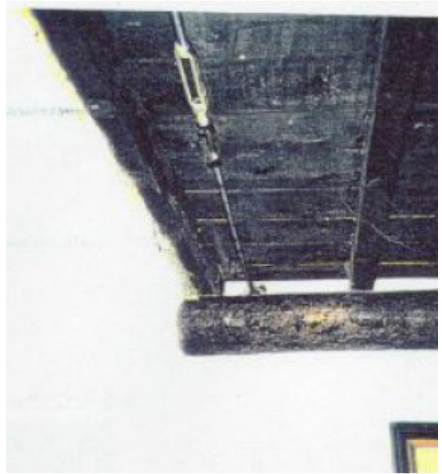
(d) Inflating the anchor with grout. (Note the photograph taken of the actual operation did not come out.)
