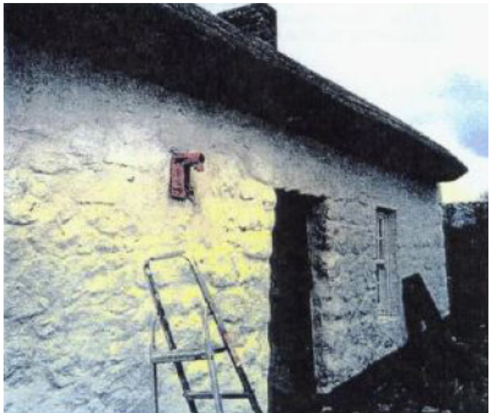
(a) Drilling Rig Base Plate fixed to wall.
