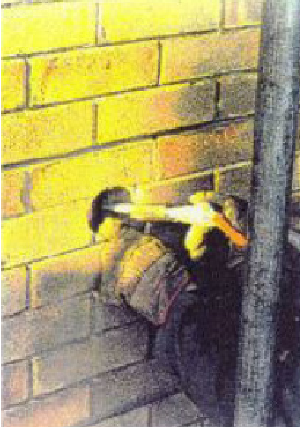
(e) Internal view of one installed anchor with the bar (connecting to the other anchor) and showing the bottle screws.
