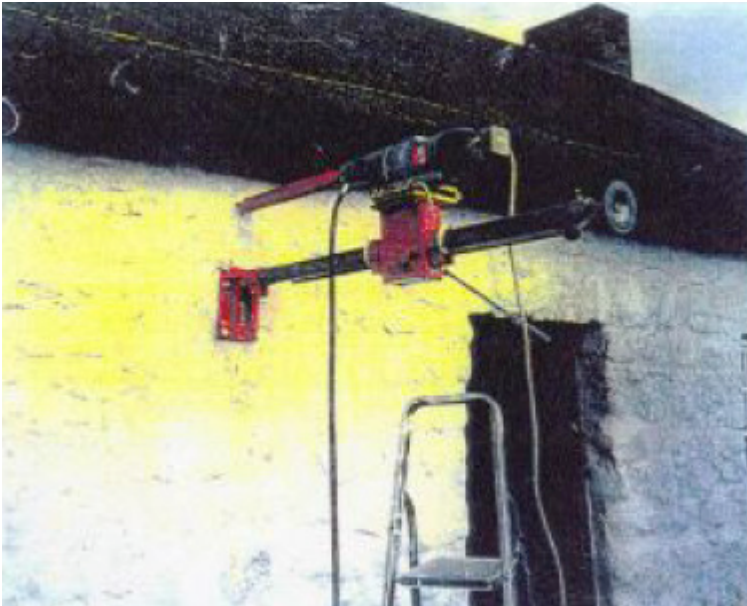
(c) Drilling one of two 60mm holes.
