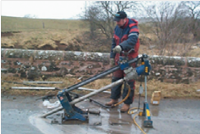
Figure 9: Strengthening in Progress
