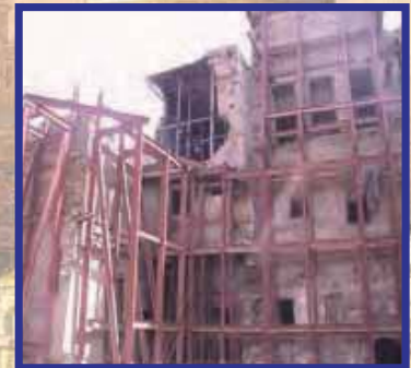
Structures with temporary supports
