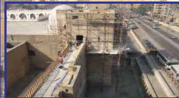
Structures with temporary supports
