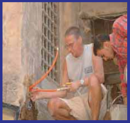
Injecting the grout from the rear to the front
