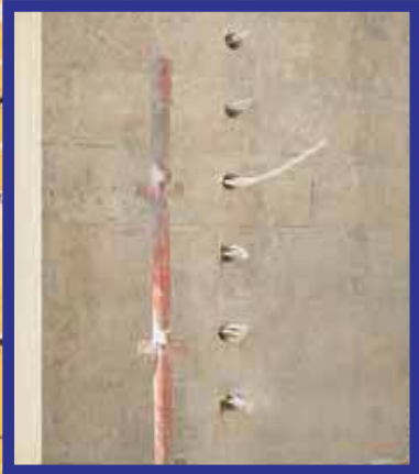
Internal cross walls stitched and secured to the external walls.
