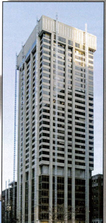
"MCWP" MAST CLIMBING WORK PLATFORM INSTALLED FULL HEIGHT
