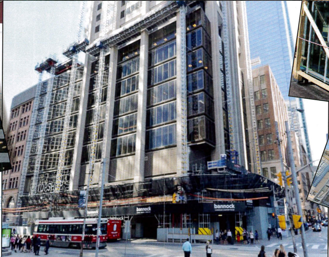
CORROSION OF ORIGINAL PANEL FASTENERS REQUIRED EXTENSIVE EMERGENCY SURFACE BRACKETING TO PREVENT PANELS FROM FALLING
