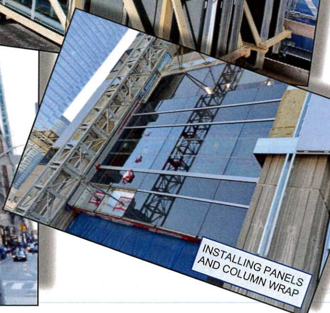
"MCWP" MAST CLIMBING WORK PLATFORM INSTALLED FULL HEIGHT
