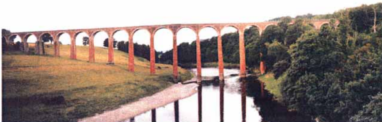
LEADERFOOT VIADUCT – SCOTTISH BORDERS
