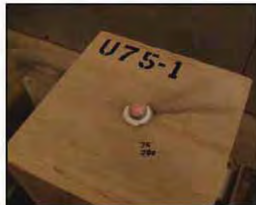
(f) Insertion of Insulation around the Rod (Silicon added to Seal the Hole)
