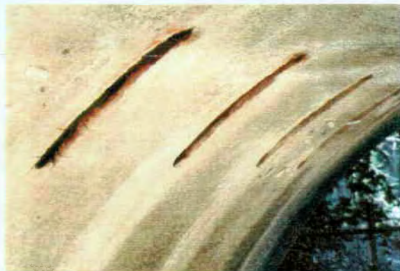
Figure 10 Installation of J-Bars
