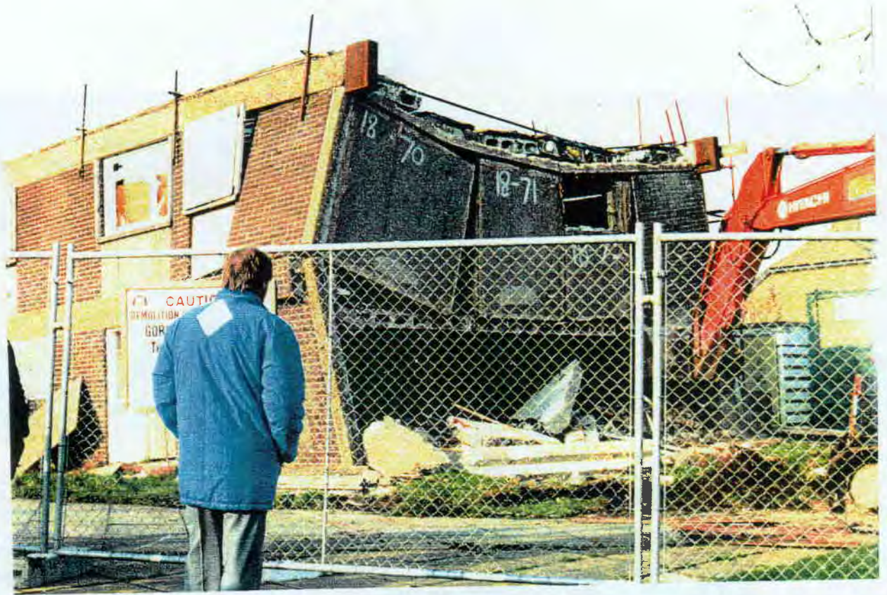
B7 As the failure progresses rapidly the roof breaks up and fails following the first floor down. Note the first floor centre wall panel is sandwiched between the roof and floor and the end is falling as a whole.
