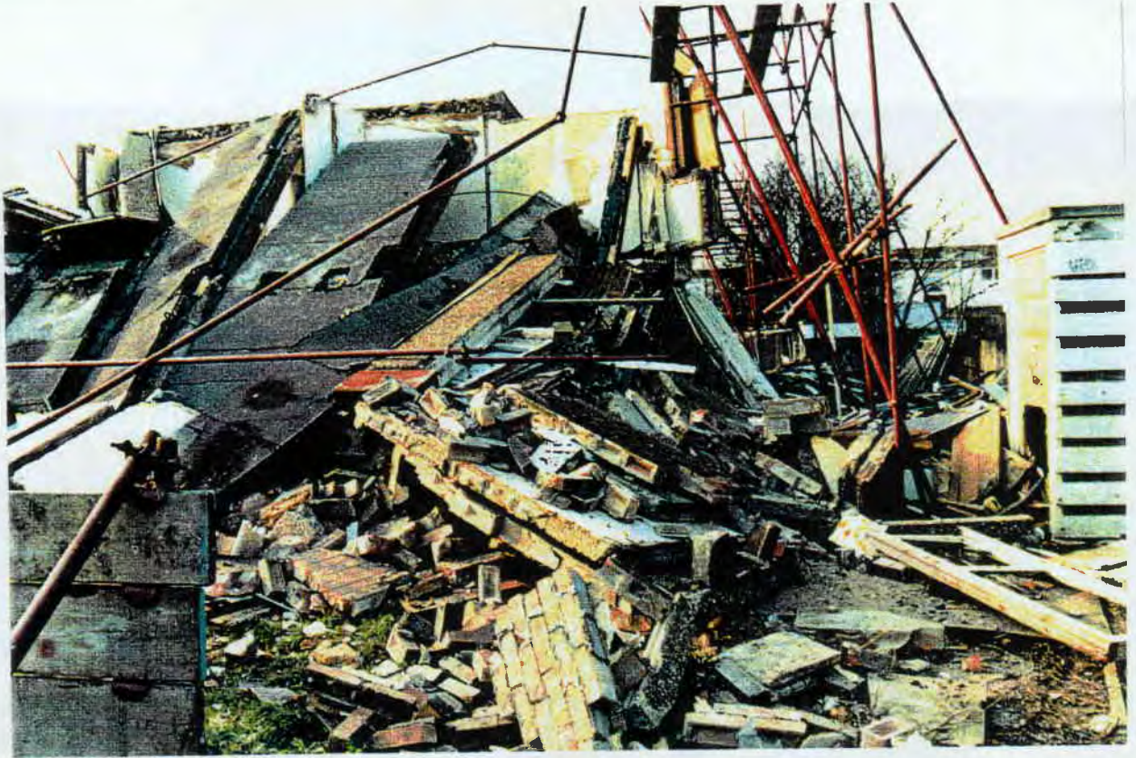
B36 Fragmented side walls had been contained by the safety scaffolding.
