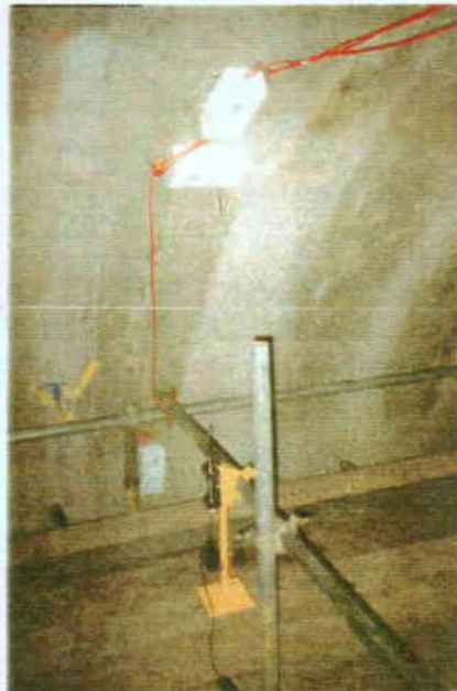
Figure 15 Deflection and Strain Instrumentation in Location
