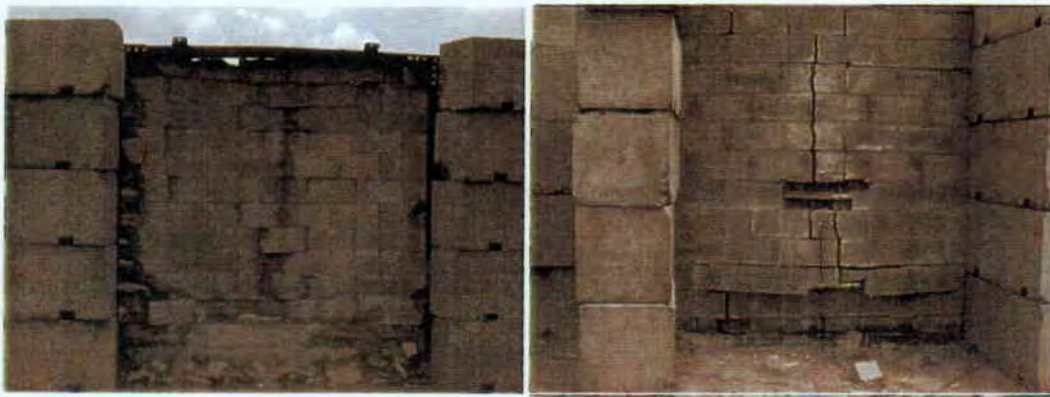
Figs 6 & 7 - Post-test photographs of the plain reinforced wall after the test: 200kg TNT NEQ @ 12.5m; 534kPa, 1274kPa-ms (440lbs TNT NEQ @ 41'; 77psi, 185psi-ms). The front view is on the left.
