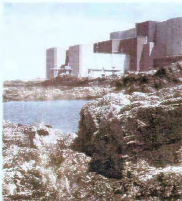
Wylfa power station, Anglesey, Wales.
