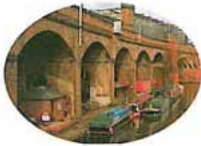
Bridge and Viaduct Reinforcement
