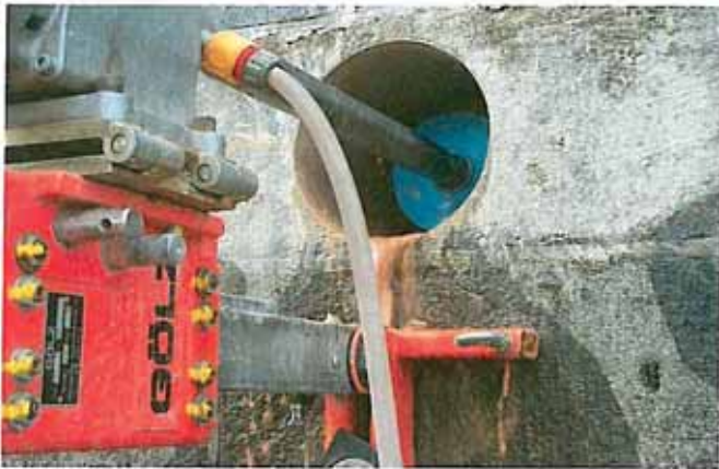
Core Drilling
