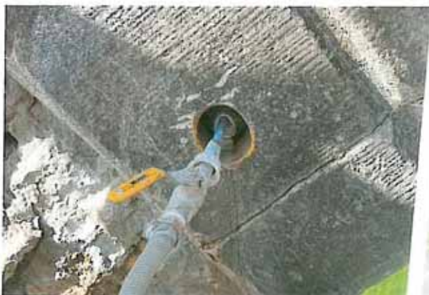
Anchor grout injection
