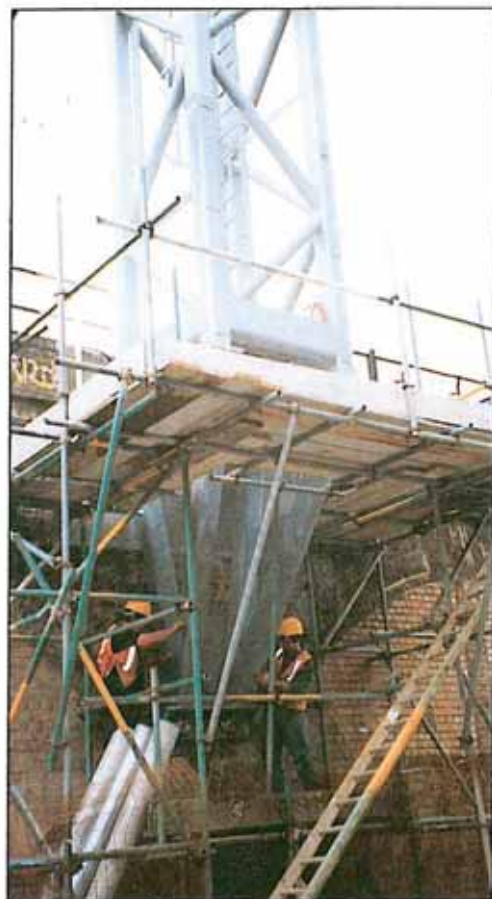
The torquing of the anchors
