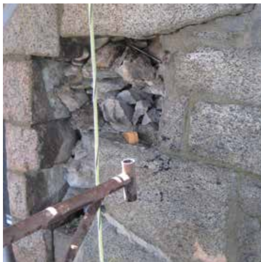
Fig. 3: Internal wall condition
