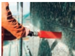
Diamond core drilling
