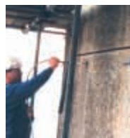
Injecting grout into anchor
