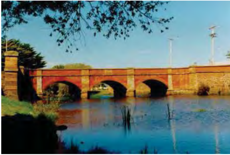
View from the west
