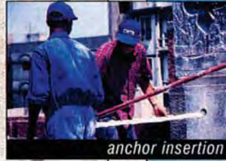
typical consolidation anchor prior to grout injection
