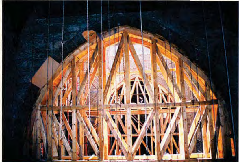
Temporary support of the Dikka arches
