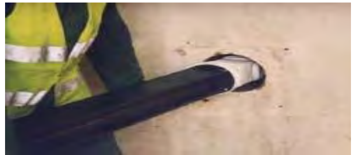
Insertion of Cintec anchor section of `I` beam into brickwork
