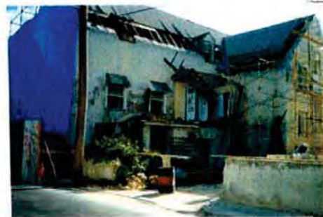
The Restoration of Arlington House [the oldest property] In Speightstown Barbados
