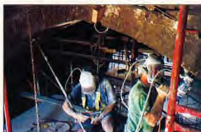
Diamond drilling the arch stones
