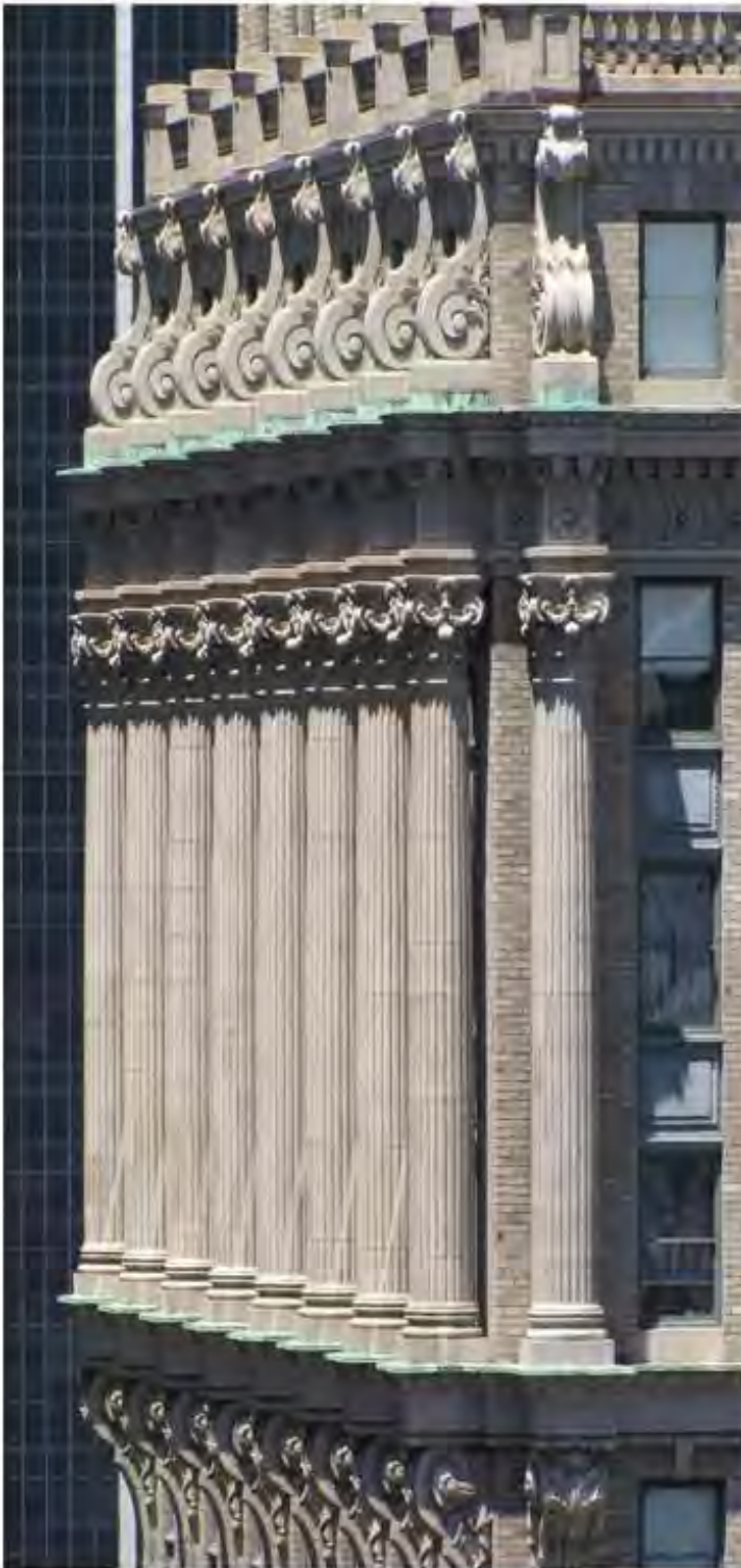
The colossal order of columns (a multi-story order of columns) is a signature feature of the building.
