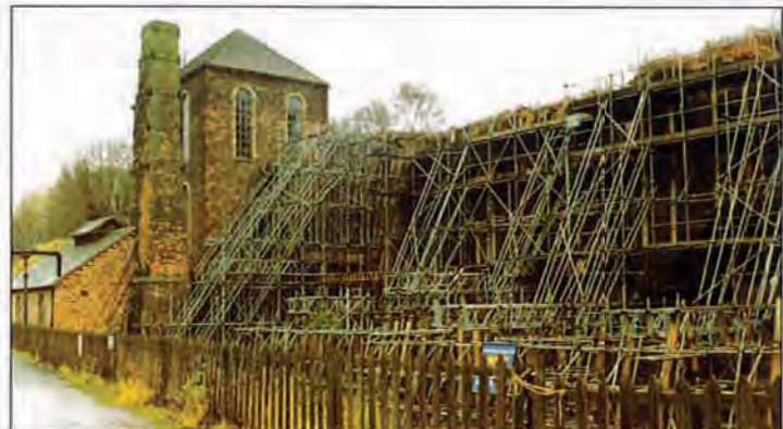
Restoration work in progress
