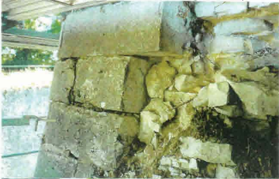
Corner, drilling for small stitching anchors, Grout mix
