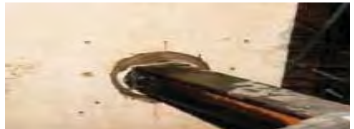
`I` beam following anchor grout injection
