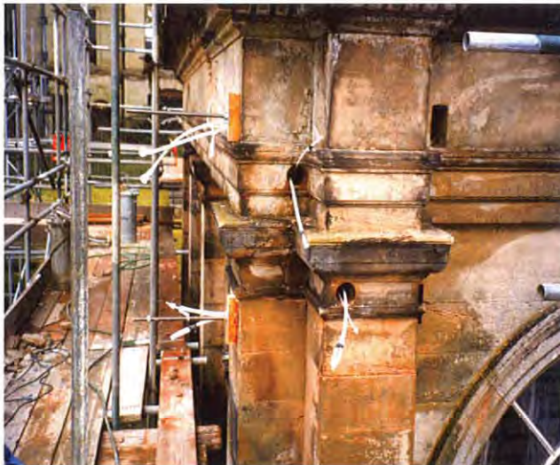
Work in progress showing the anchors positioned and inflated prior to making good and cleaning
