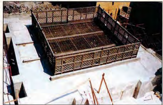
Roof section above central courtyard
