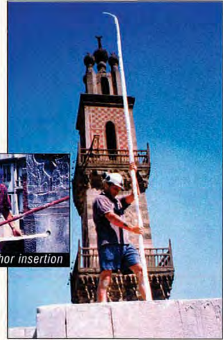
5 metre long vertical anchors at roof level
