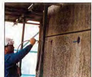
Injecting grout into anchor
