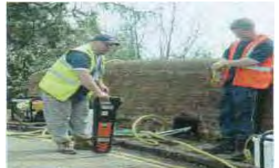
Checking for sub-surface services during bridge survey
