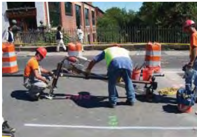
Workers bolt the drilling rig to the pavement on the bridge in preparation for drilling the 26 holes needed for the strengthening project.
