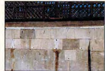
Roof consolidation anchors
