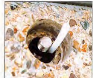
Anchor prior to injection
