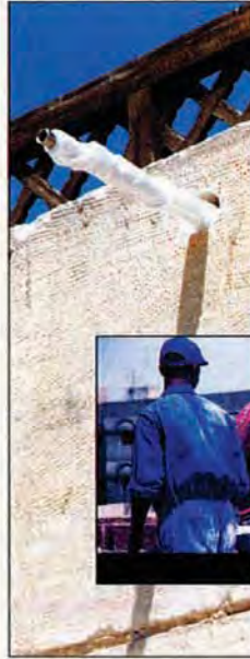
typical consolidation anchor prior to grout injection
