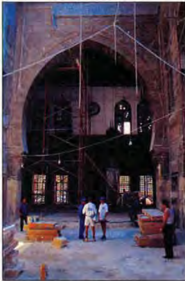
Dikka arch in the main courtyard
