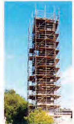
Chimney Restoration In Progress
