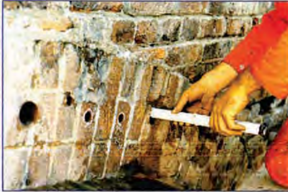
Placing the anchor in the prepared hole
