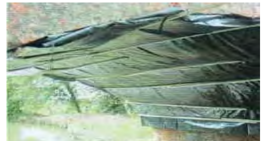
Temporary below arch protection during the installation process
