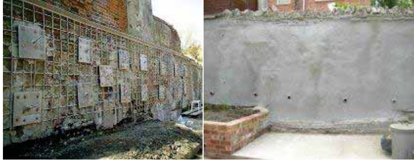
Mesh and face plates secured.....Final lime rendered finish applied
