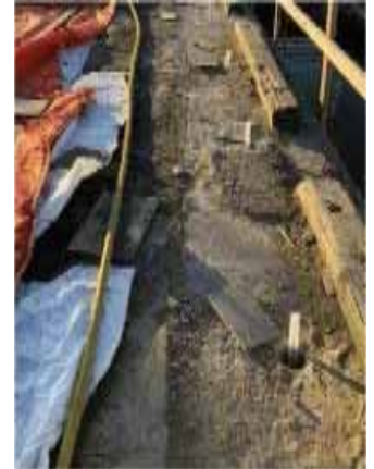
Cintec anchors in place prior to inflation
