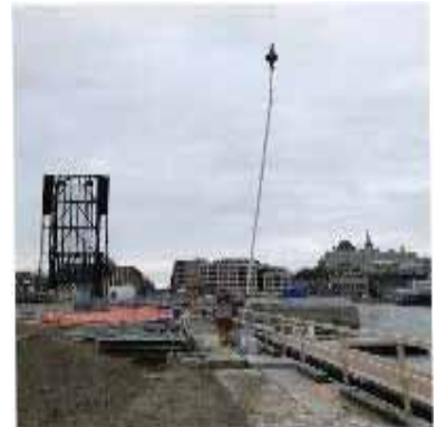
Cintec anchors being lifted into place Quebec Canada
