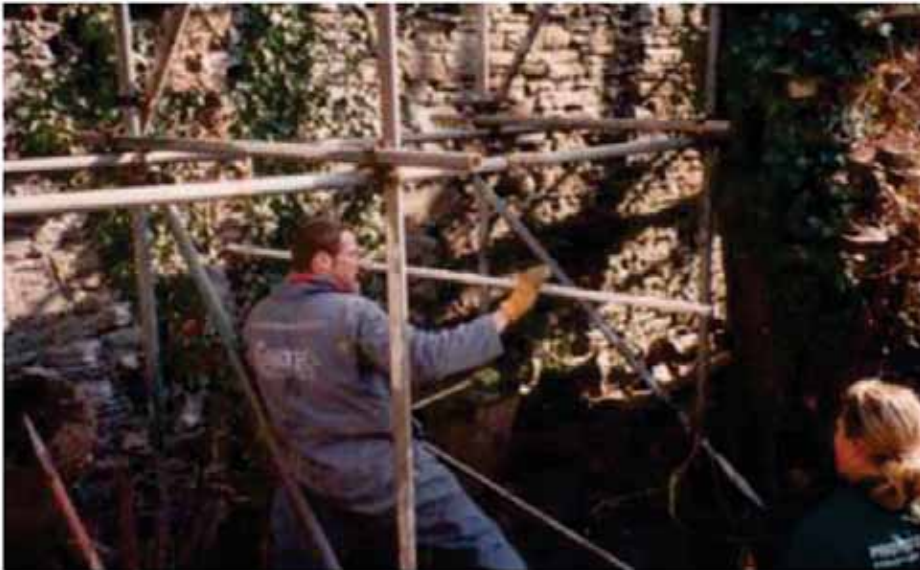
Insertion of 3m Cintec Anchor (left). Its inflation using cementitious grout, (above).
