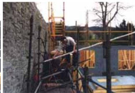
Carefully placing the anchor
