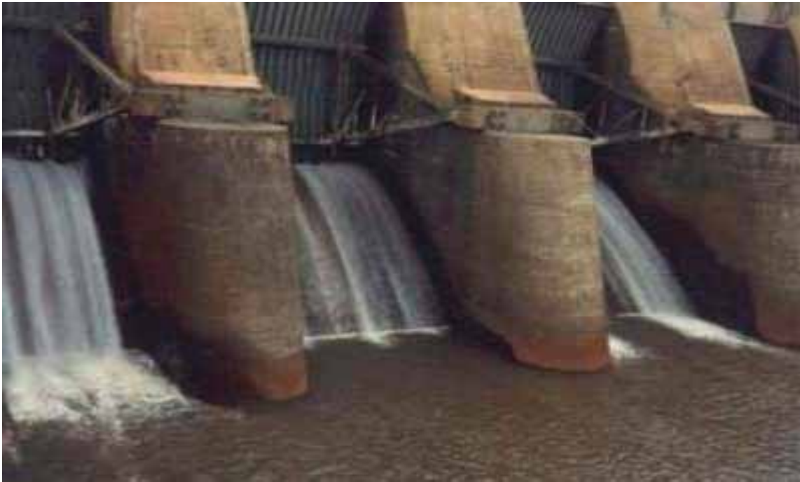
Hydro-Electric Dam repairs Nigeria
