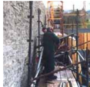
Adding mining barrel extensions
