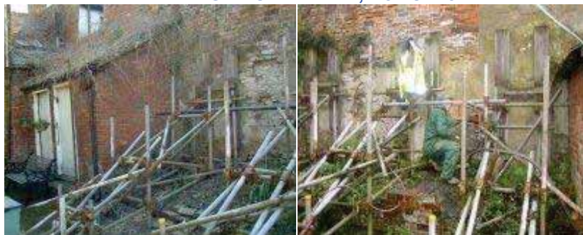
As found shored up .....Drilling and installing Cintec ground anchors
