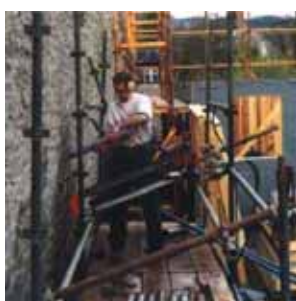
Extracting the tube liner
