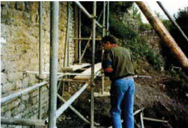
Diamond drilling (right) and anchor insertions (left).
