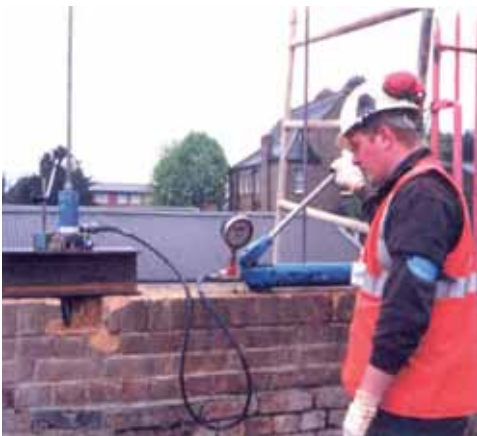
Post-tensioning Cintec anchor in test panel.
