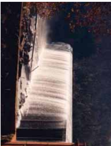
Georgia-Power Bartletts ferry dam, Athens, Georgia, USA
