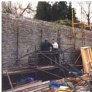
Setting up the drilling rig
