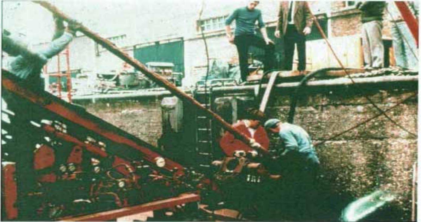
Strengthening of Zeebrugge Harbour Wall (Belgium)
