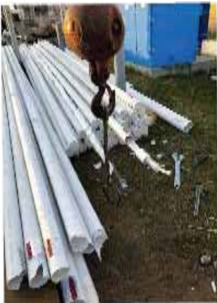
Cintec anchors in protective shipping tubes
