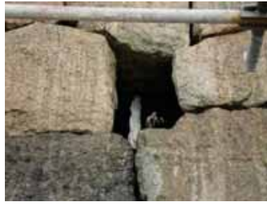
Pre-injection with masking tape
