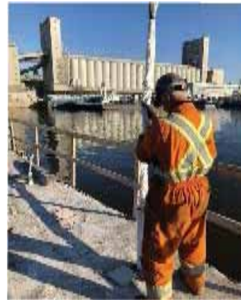
Cintec anchors being placed by installer
