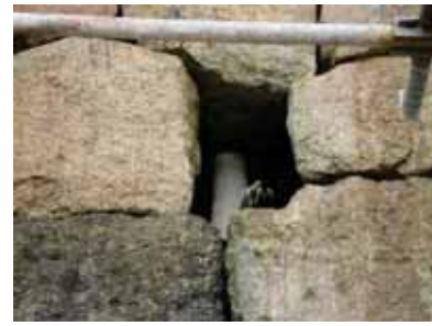
Anchor grouted & expanded
