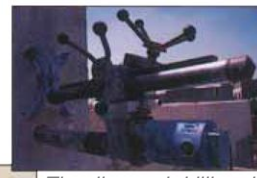
The diamond drilling rig
