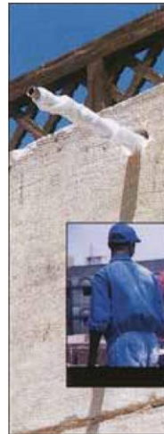
typical consolidation anchor prior to grout injection
