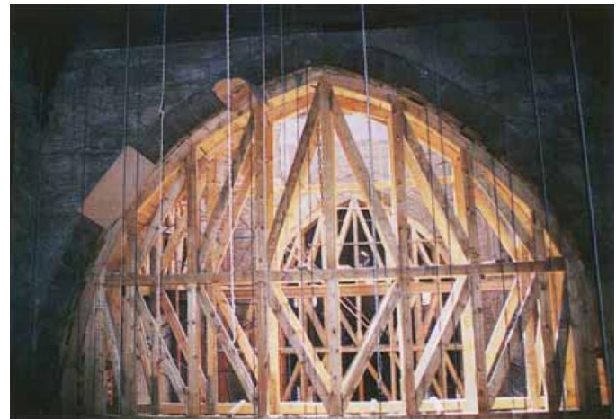
Temporary support of the Dikka arches
