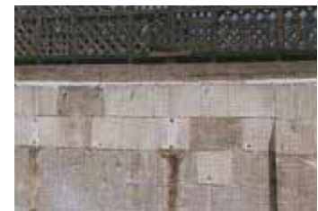
Roof consolidation anchors
