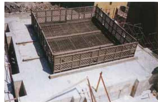
Roof section above central courtyard
