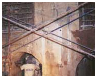
Drilling the vaults
