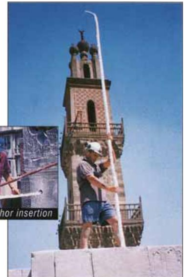
5 metre long vertical anchors at roof level
