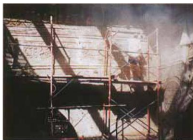
Decorative panels being drilled ready for installation of consolidation anchors
