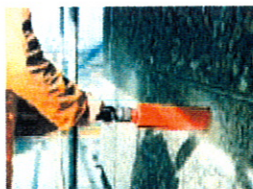
Diamond core drilling
