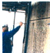
Injecting grout into anchor
