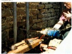
The anchors were installed through the joints of the stonework following the completion of gravity grouting of extensive voids within. To facilitate this process, clay was used to seal the open joints between the stones in order to retain the original historic grouting. This was later removed and the wall pointed with lime mortar to match the original material. The Cintec ground anchors were tested to a working load of 15kN. Other, smaller Cintec anchors were also used for wall consolidation.
