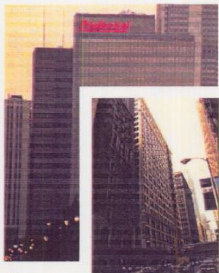
The Prudential The Chicago Building Jewellery Exchange
