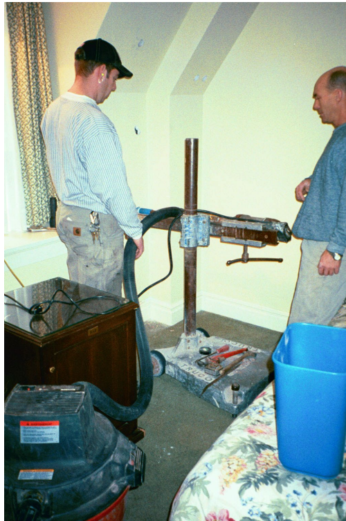
Dust – free Directional Drilling
