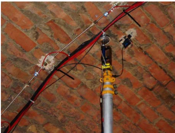
b. Typical crack and displacement LVDTs
