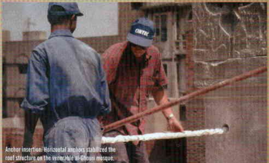
Typical anchor placement for the arches and side walls.
