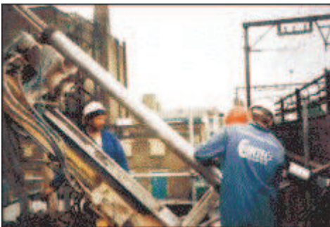
The assembling and installation of a compression anchor
