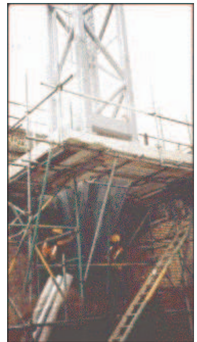
The torquing of the anchors
