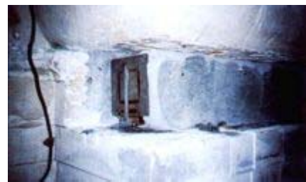
Beam after grout injection
