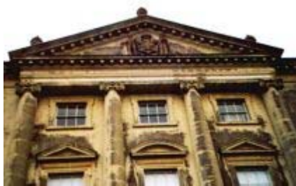
External upper beam area
