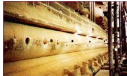
Anchor installation
