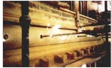
Drilling & securing stonework above beam
