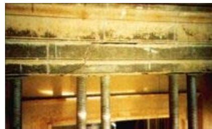
First sign of distressed beam
