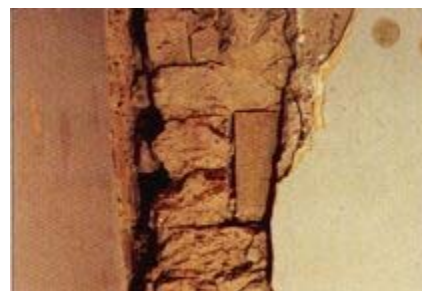
Internal damage of wooden beam
