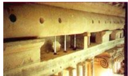
Entire length of 10 metres exposed
