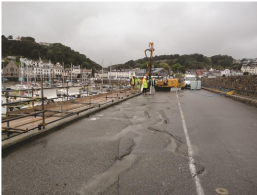
North Pier - cracks at deck level
