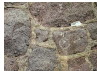
Figure 20 - Anchor with plug cap replaced, 'Secret Fix'
