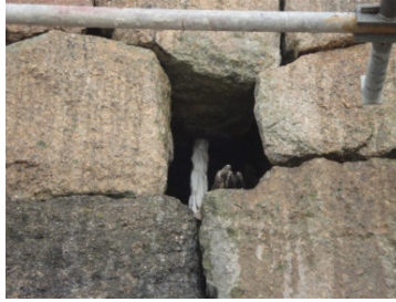
Figure 16 - Pre-injection with masking tape
