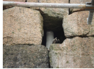
Figure 17 - Anchor expanded
