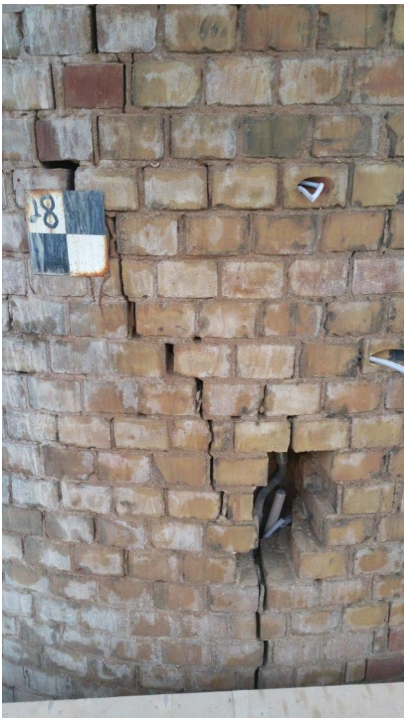
All cracks were stitched horizontally with M16 stud anchors in 40mm holes.
