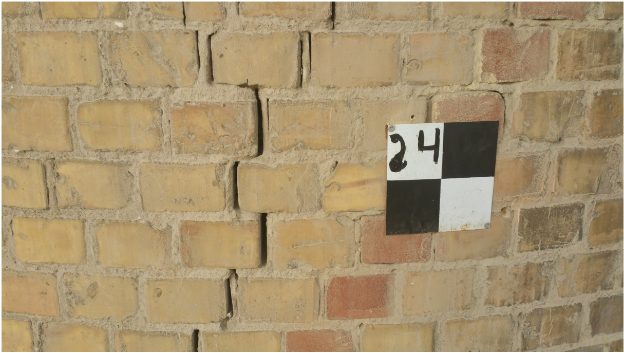
All cracks were stitched horizontally with M16 stud anchors in 40mm holes.
