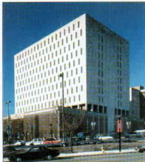
Limestone cladding of Essex County New Courts Building and Jail was one accident away from catastrophic failure. More than 20,000 Cintec anchors now prevent masonry's collapse.
