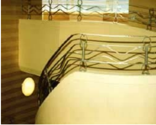
One of the two Cintec Anchor supported stairwells fully renovated.
