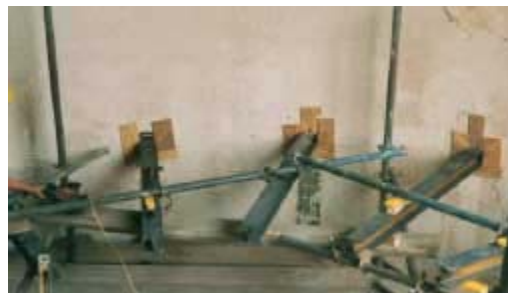
All installed 'I' beams leveled and supported as grout hardens
