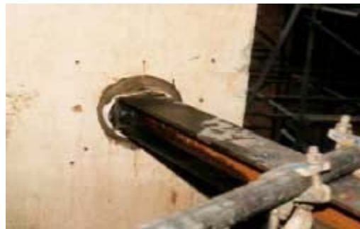
'I' beam following anchor grout injection
