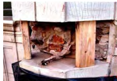
Fig. 2 - Corroded restraint fixing
