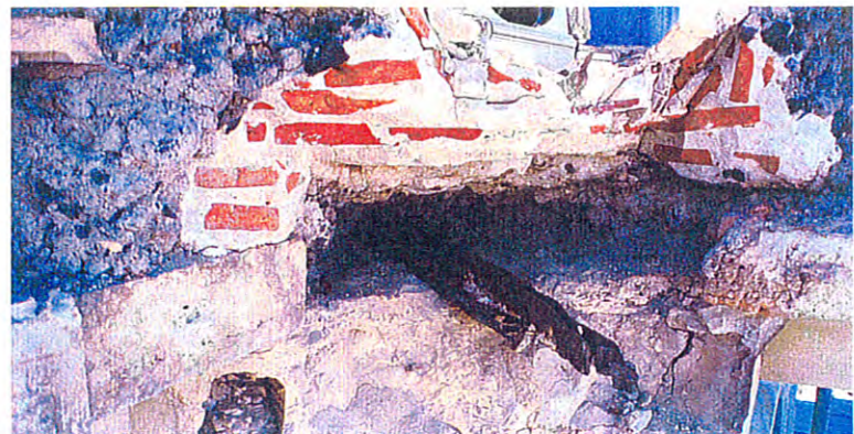
Once the cornice had been partially disassembled, the materials and techniques used in its construction could be easily identified. Note the clinker concrete, or "cindercrete," between the terra-cotta blocks and the brick backup material, and the severe deterioration of the steel supports. CSI recommended that all new steelwork be AISI Type 516 stainless steel, a non-corroding type, which is essential in this chloride-rich maritime environment.
