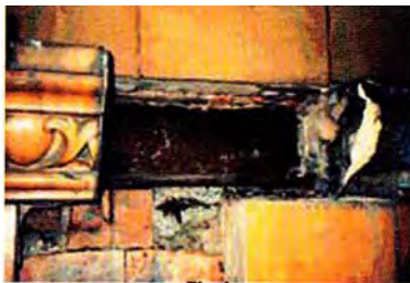
Fig 1 Example of steel beam corrosion causing failure of the decorative terra cotta facade.
