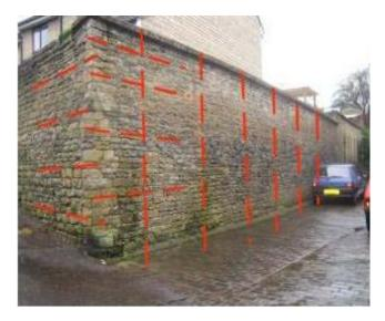
Engineers Mann Williams devised a scheme to save the situation by installing Cintec ground anchors through the wall at one-third height together with vertical Cintec anchors to reinforce & mobilize the full height of the wall to resist the rotational effect. Anchors were located as shown by dotted red lines.
