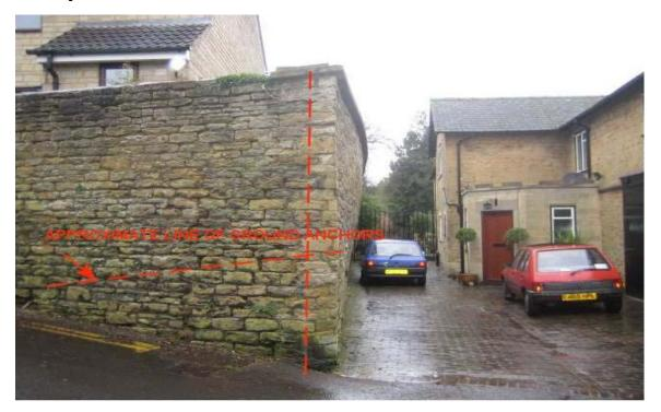
AS can be seen from above photograph this retaining wall has seriously rotated towards the next property. Understandably the neighbors were becoming extremely concerned about its safety. The wall retained the garden and some imposed load from the house foundations.
