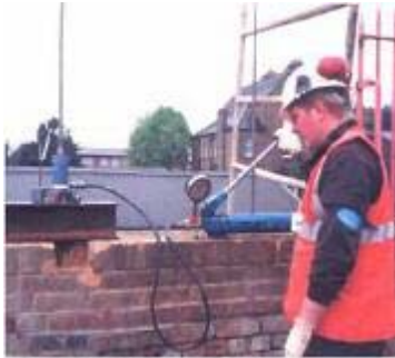
Post-tensioning Cintec anchor in test panel.
