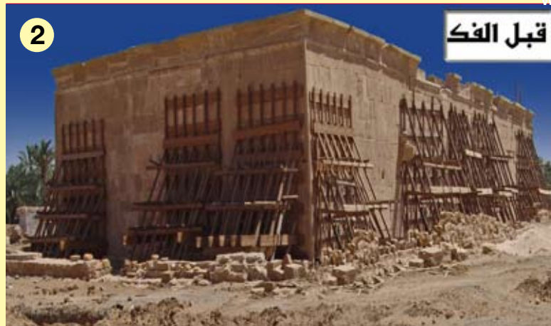
(2) The original, supported corner
