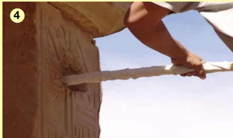
(2) Drilling for the Anchor (4) Inserting the CINTEC Anchor
