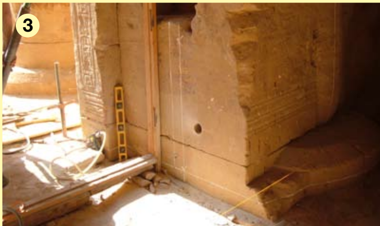
(1) Securing the Ground (3) The finished hole ready for the anchor
