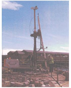
A mobile rig was employed firstly to core drill the anchor holes, then to temporarily install a metal tube hole lining, following by the lifting and lowering of the Cintec anchor (above) and finally the removal of the temporary core lining prior to anchor injection
