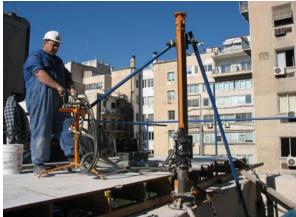
The dry drilling used compressed air as the cooling and flushing medium. Heavy duty vacuum extractors were used to minimise dust levels, both internally and externally.
