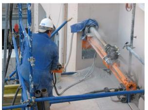
Horizontal holes were dry drilled through hard limestone random rubble walls using 86mm core barrels on lengths up to 10mts and 101mm core barrels for the longer lengths, these were reinserted after drilling to facilitate the anchor installation.
