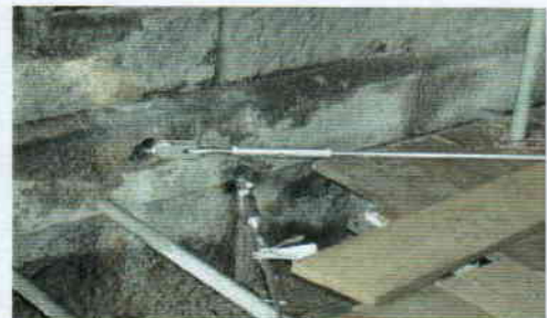
Lower fixing detail with turn buckles.
