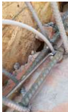
Figure B show the installed anchors with wire cage.
