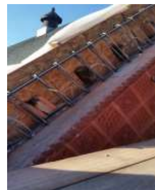
Figure C is the wire cage attached to the terra cotta along the full length of the gable end.
