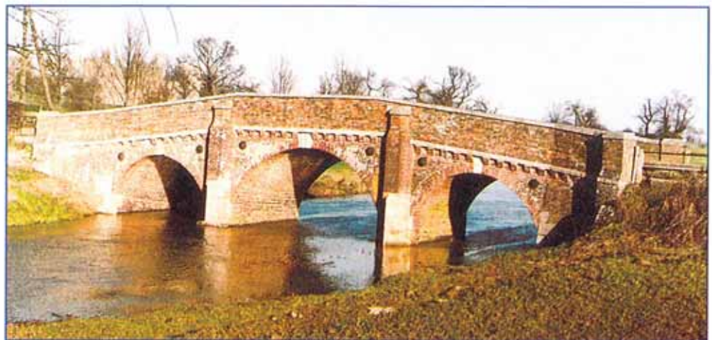
Bodiam bridge after completion with the castle behind the trees in the background.
