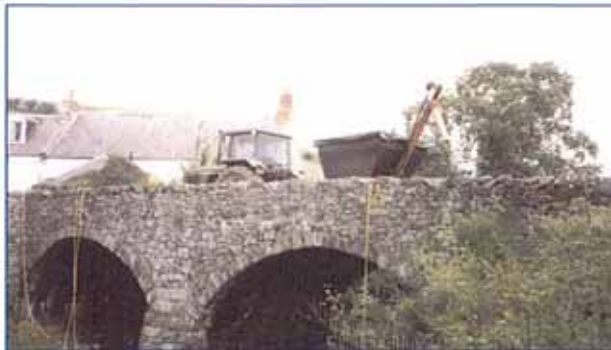
CLIFTON BRIDGE - SCOTTISH BORDERS
