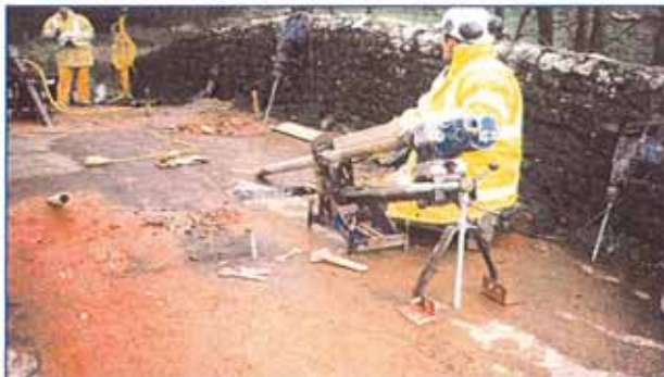
AMBERSHAM BRIDGE - WEST SUSSEX
