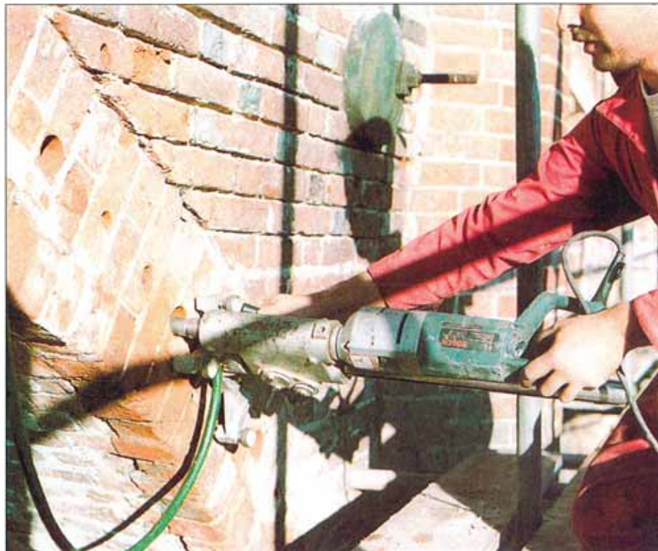
Core drilling holes for the anchors
