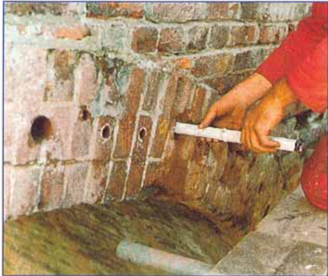
Placing the anchor in the prepared hole
