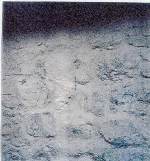
(g) The finished wall after installation of anchor and before white washing.
