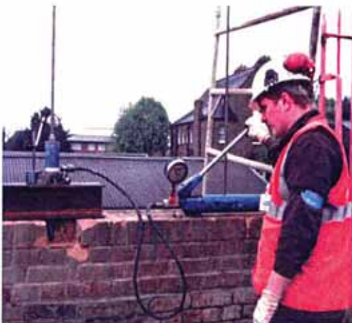
Post-tensioning Cintec anchor in test panel.
