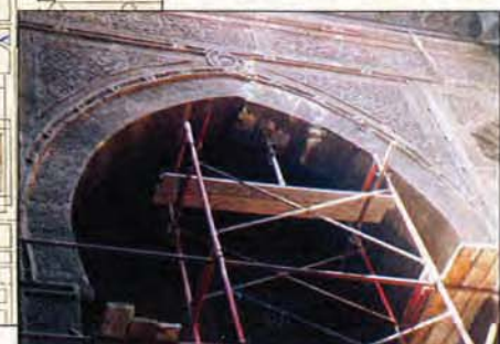
One of the four arches of the court being scaffolded prior to drilling and anchoring
