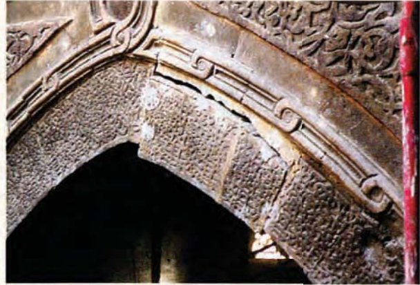
Seismic damage to decorative arches
