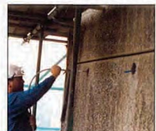
Injecting grout into anchor
