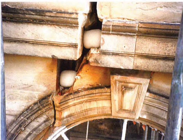
Work in progress showing the anchors positioned and inflated prior to making good and cleaning
