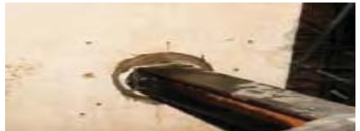
'I' beam following anchor grout injection
