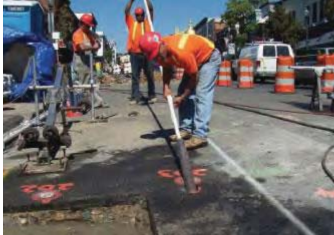
Workers insert the fabric sleeve and stainless steel reinforcing rod into the drilling pipe, which is later removed. In the background, traffic continues to move across the bridge during the work.
