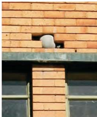
Anchor being inserted in protection sleeve in cavity – sleeve later removed
