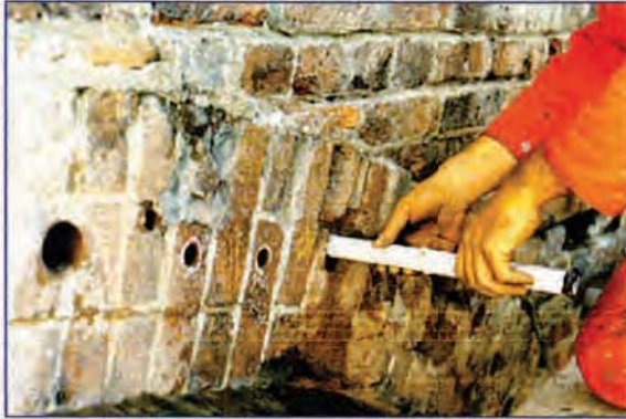
Placing the anchor in the prepared hole
