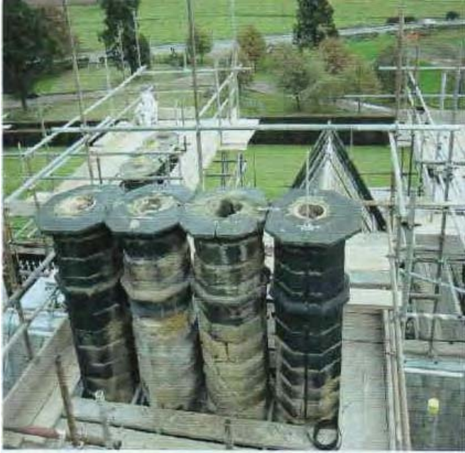
Partially missing ceramic liner ->
