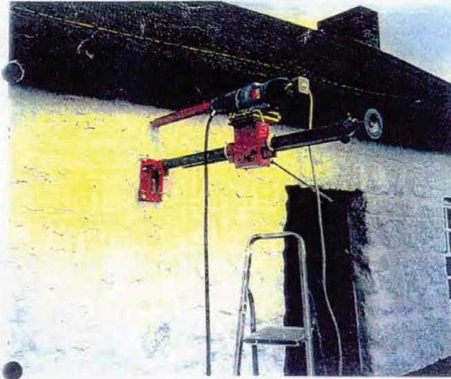
(b) Drilling Rig in place.
