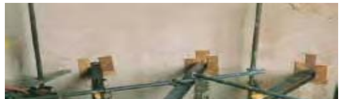
All installed 'I' beams leveled and supported as grout Hardens
