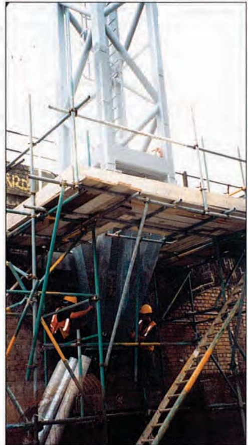
The torqueing of the anchors
