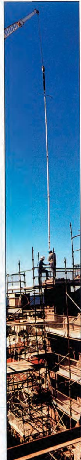
20 m vertical anchor being placed by crane in the project which saw anchors up to 32 m horizontally, Cintec's longest to date.
