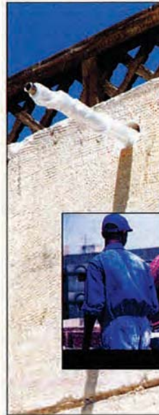
typical consolidation anchor prior to grout injection
