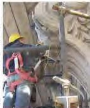
Grout being pumped into the terra cotta anchor assembly to engage and stabilize terra cotta units.
