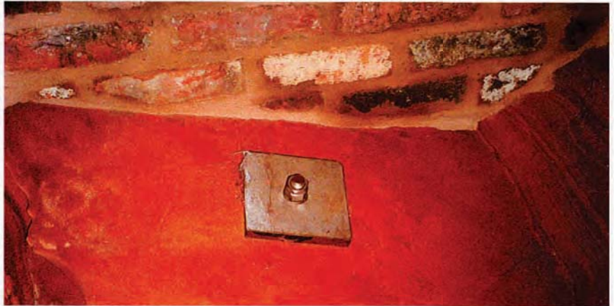
Roof bolt support to ballroom ceiling.
