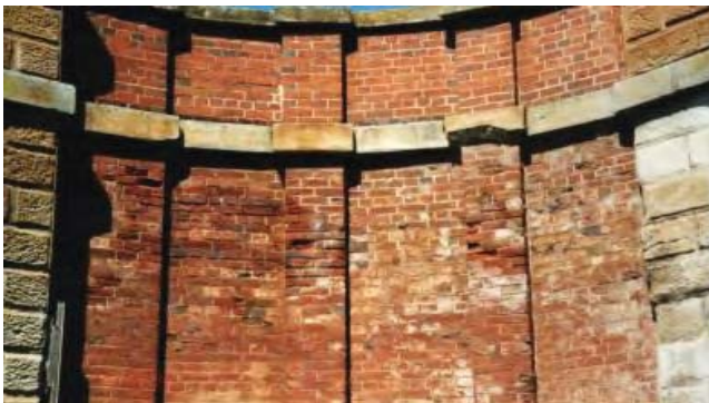
Damage to wingfall – note coloured cement render from 1930's and salt deposition caused by it
