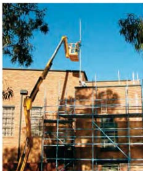
Anchor being inserted in protection sleeve in cavity – sleeve later removed
