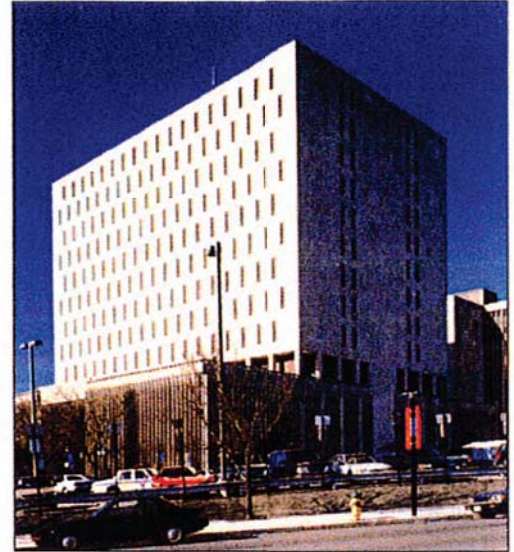
Limestone cladding of Essex County New Courts Building and Jail was one accident away from catastrophic failure. More than 20,000 Cintec anchors now prevent masonry's collapse.
