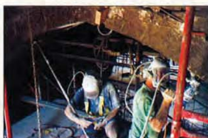
Diamond drilling the arch stones
