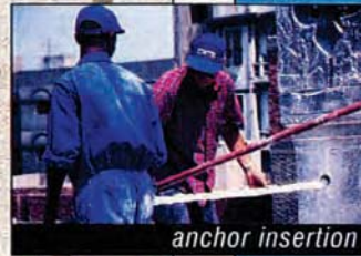
typical consolidation anchor prior to grout injection
