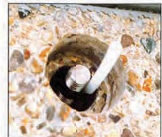
Anchor prior to injection
