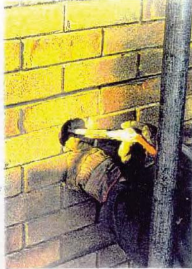
(e) Inflating the anchor with grout. (Note the photograph taken of the actual operation did not come out).
