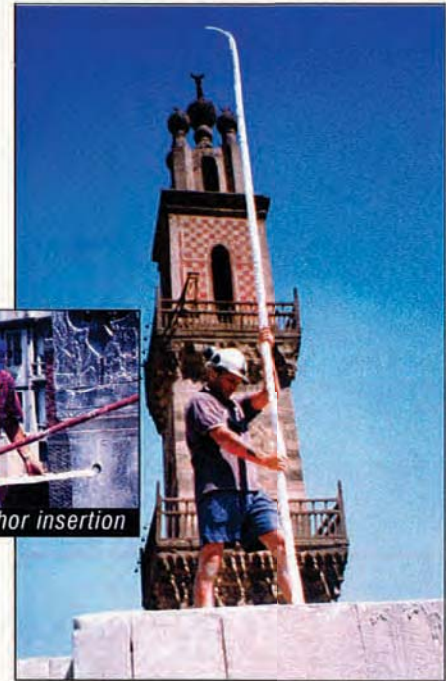
5 metre long vertical anchors at roof level
