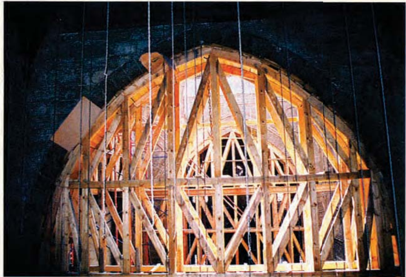
Temporary support of the Dikka arches
